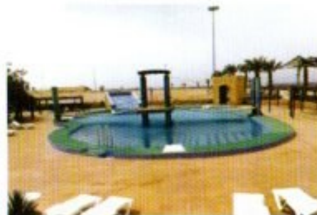
Pipeless Filter in JORDAN
