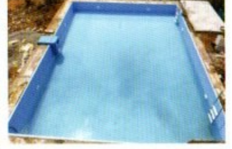
Liner Renovated Pool with PLF at HYDERABAD
