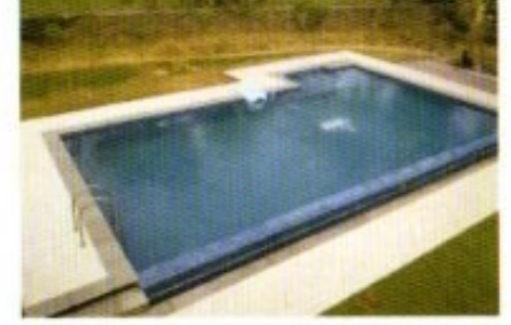
Pipeless Filter in Infinity Pool
